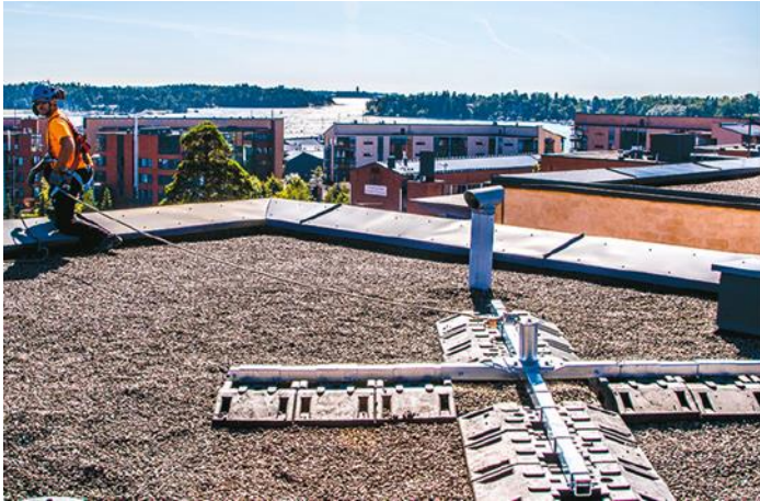
1. Counterweight anchor, weight 374 kg
